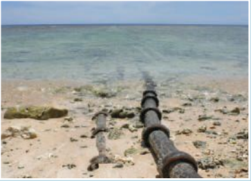
The Gun Beach conduit in Guam
